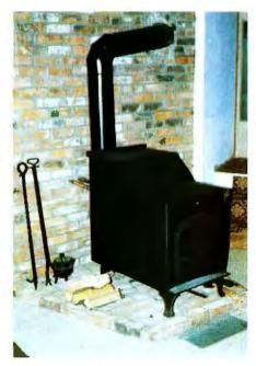
**Photo 1:** The Hydrostove is installed in the corner of the Circuit Cellar. Take note of the two copper pipes coming out the rear of the stove into the wall. The pipes, which are buried behind the wall and above the ceiling, go to the furnace, which is 35 feet away.
