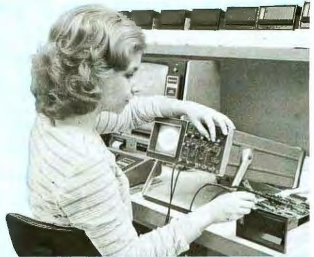
"Connie is running a 'cats eye' test on a mini-disk drive to check radial track alignment. Drive motor-speed timing and sensor alignment tests have already been performed. Disk formatting and format verification tests are next. These measurements are part of the 100% testing every single unit receives."
