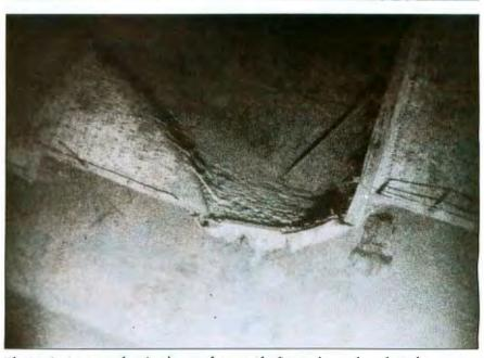
Photo 4: An area of major damage between the first and second smokestacks.
