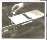
Nex1, you install the disk drive. You learn disk drive operation and adjustment, make a copy of the MS-DOS operating disk, and begin your exploration of the 3088 CPU.
