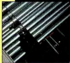
Jason Frand (above) spearheaded a technology program for UCLA's Anderson School. Cables are pulled through individual conduits for easier upgrading (inset).
