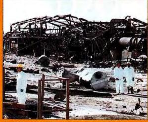
In 1988, a series of explosions, the largest one exceeding the equivalent of 1.5 million pounds of TNT, destroyed a chemical plant in Henderson, Nevada. Two people died, and the surrounding community suffered more than \$70 million in damages. Fallure **Analysis determined** that the explosion was due to a leak in a natural-gas line under the plant.
