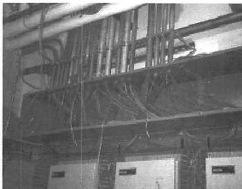
Feeder Tubes, Cables, and Junction Box
