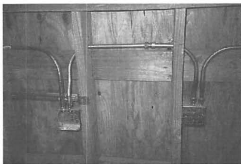
Two Gang Boxes Daisy-Chained Together
