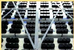
Lead gel batteries guarantee continuous power without interruption.
